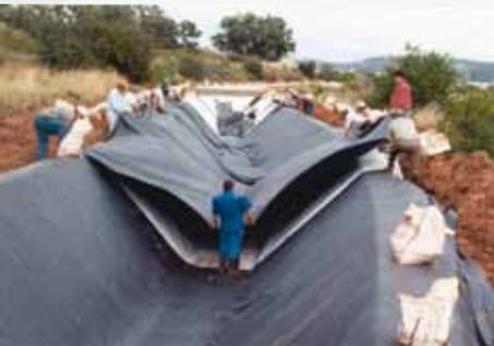
Firestone EPDM Geomembrane is an elastomeric synthetic rubber membrane with a cross linked polymer structure resulting in a chemically stable membrane with unique features and benefits.
