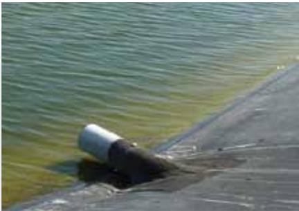
Flashing of pipes, other penetrations, inside and outside corners is fast and easy with use of Firestone QuickSeam FormFlash, an uncured EPDM flashing laminated to a self-adhesive QuickSeam Tape. It can be easily molded to adapt to any shape.
